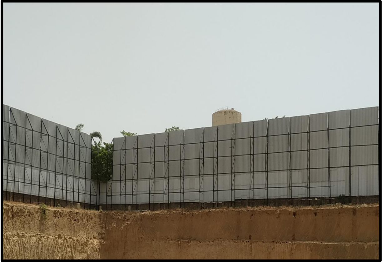
Inside - Rear Road Barricading
